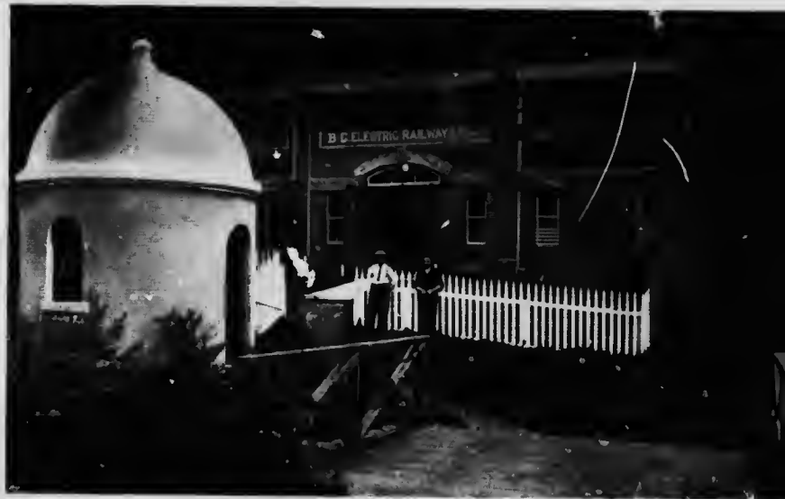
British Columbia Electric Railway Company, Limited. Goldstream Power House.
